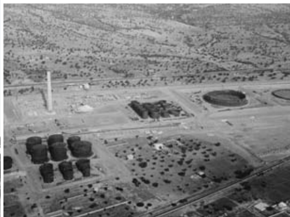
The stack and two groups of tanks under construction. Centre right - a large crude oil tank is beginning to take shape (1971)
