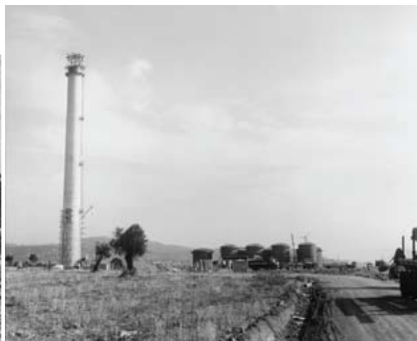
The lubricants refinery stack under construction (1971)
