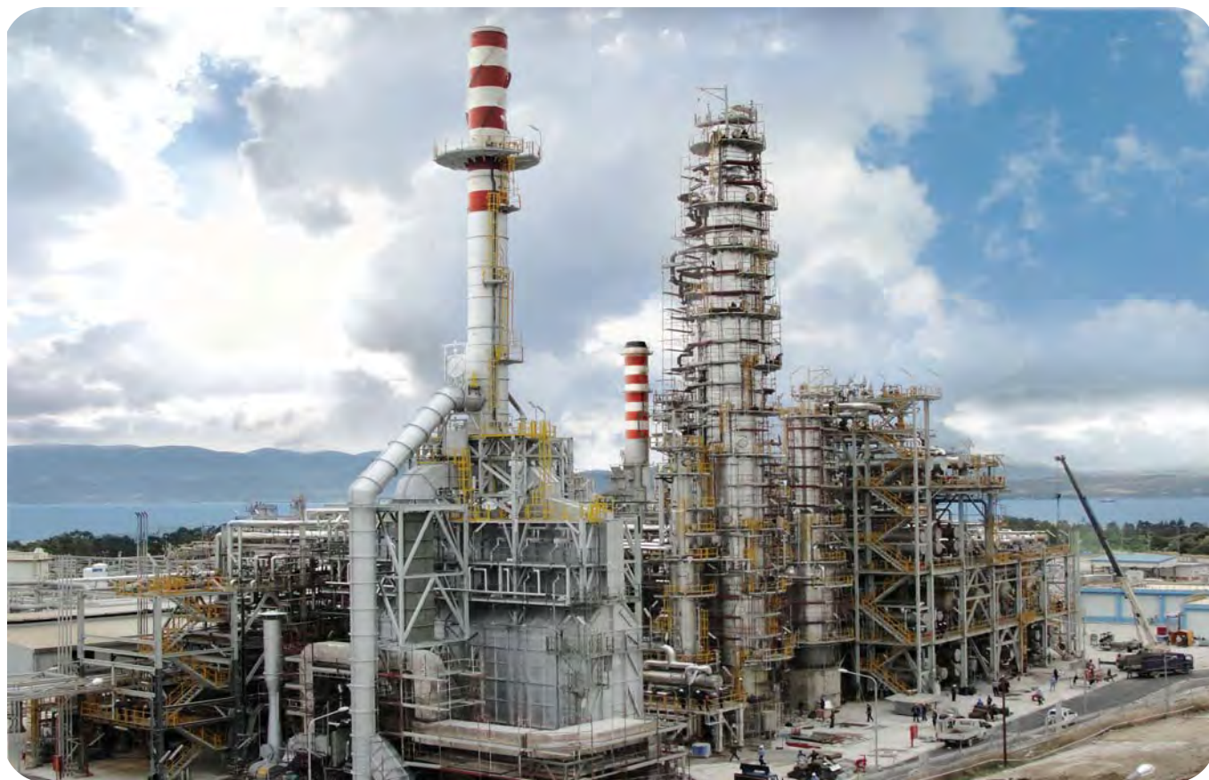
The new Crude Distillation Unit at the final construction stage.
