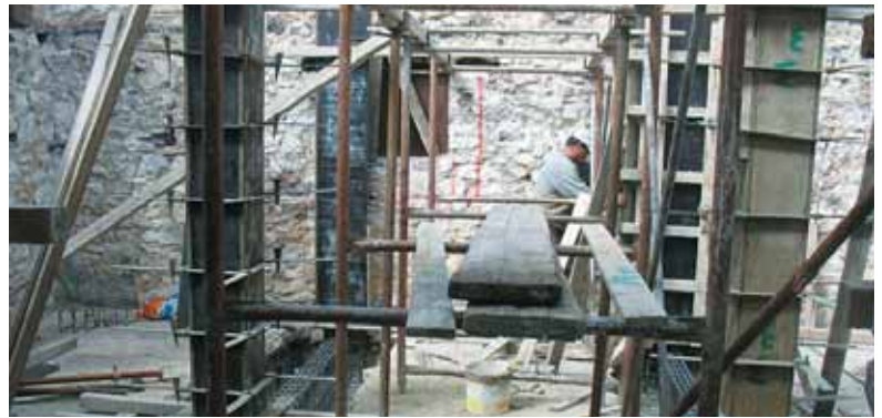
View of the repair works on a home.
